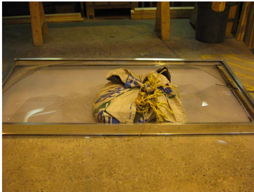
Photo No. 2 Curb Mount Skylight Failure
